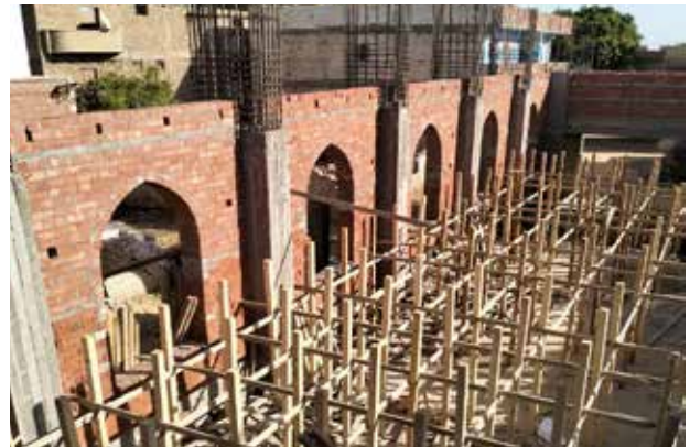
Tenth of Ramadan New Church, The Framework Is Completed
