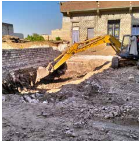
Church buildings under construction
