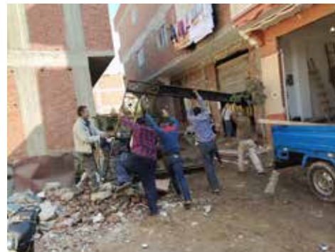
2 buildings under construction
